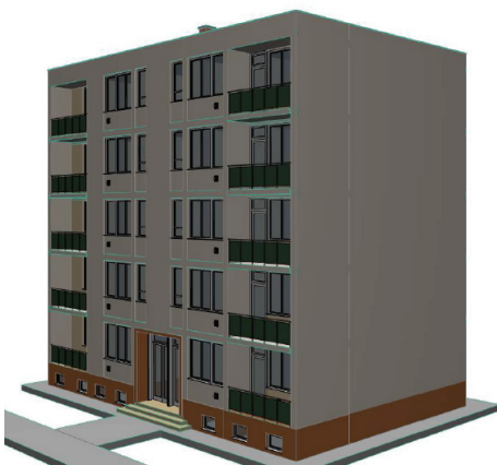
Fig. 2. Multifamily house built with traditional technologies
