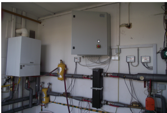
Fig. 1. Heating system of the Building Mechatronics Research Center
