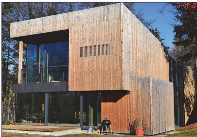
Fig. 1. Sibelius Solar house, front and back overview
