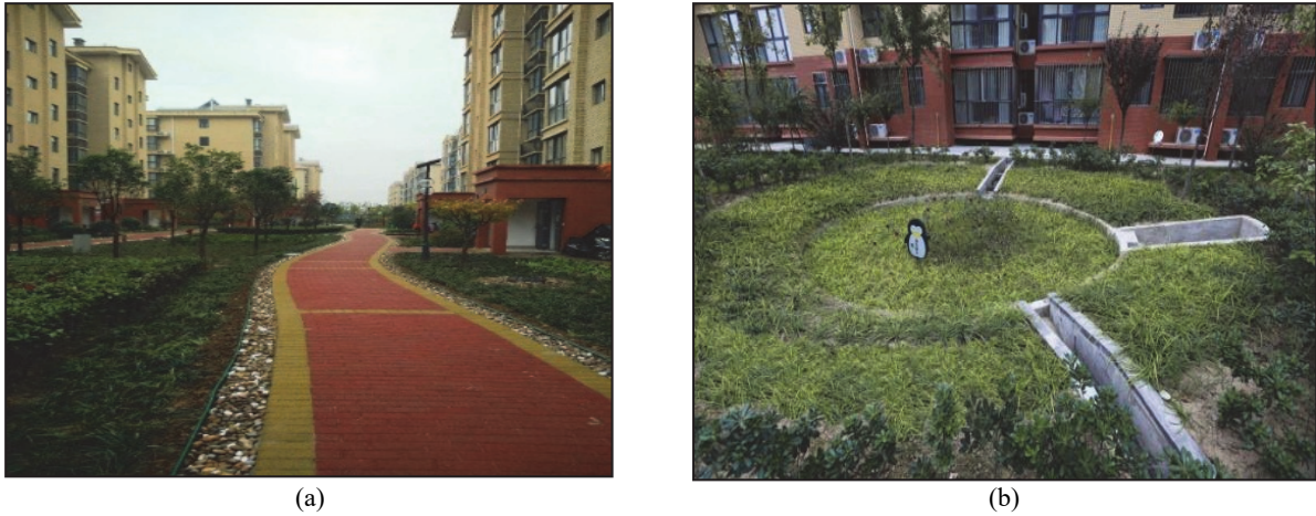
Fig. 2. LID measures: (a) Permeable pavement, (b) Rain garden
