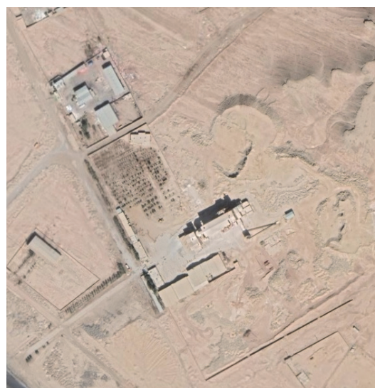
Fig. 1. Aerial view of Zarch Gypsum plant (Reproduced from Makermi et al. (2019), under the terms of Creative Commons Attribution 4.0 International License)
