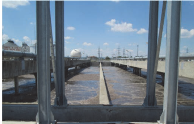
Fig. 4. Iasi WWTP – Bioreactor no. 2
