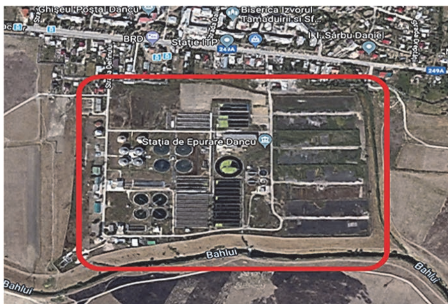
Fig. 1. View and site of the Iasi wastewater treatment plant
