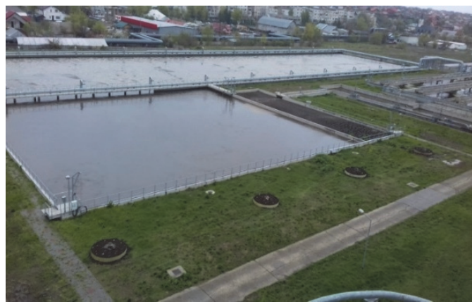
Fig. 5. Iasi WWTP – Bioreactor no. 3
